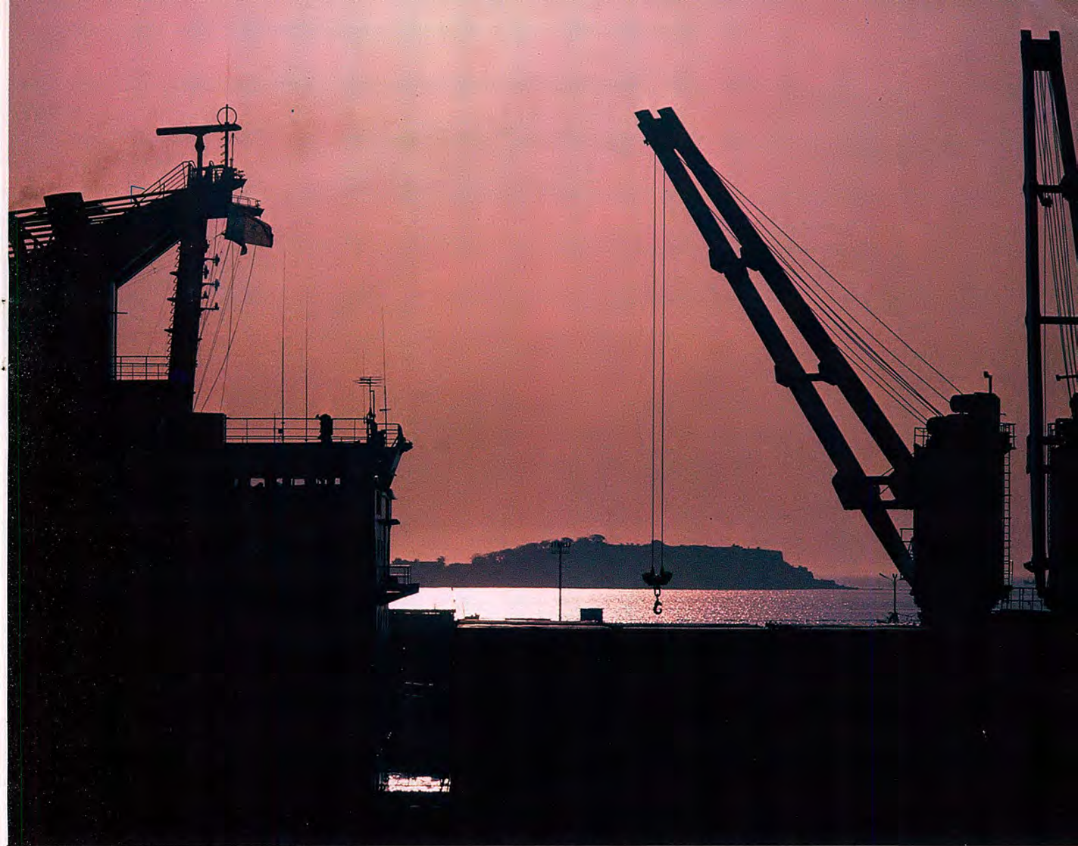
Dakar harbour, Senegal, is well equipped to handle containers which carry raw materials and semi-manufactured goods to overseas markets.
